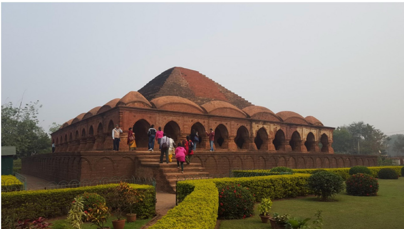
Front view of the Rasmancha temple
